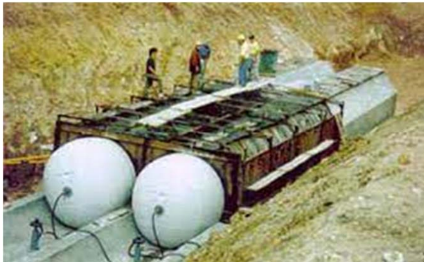
Fig 4. Tubular inflated formwork for the construction of water lines [8]
